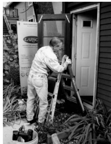
Bob Balderson installing new storm door
